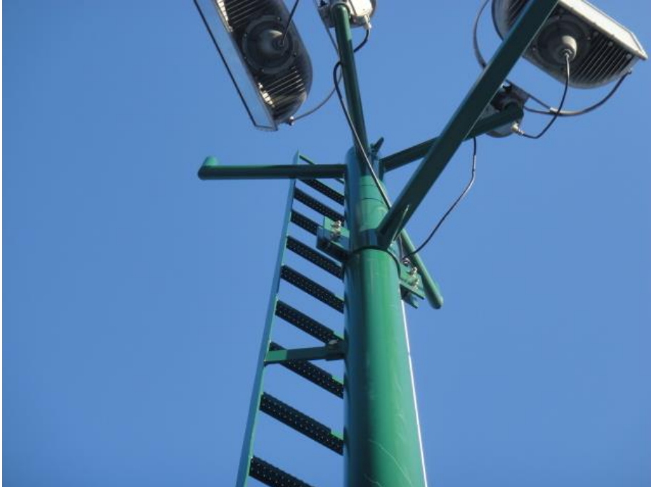
Intermediate Tower Idler Wheel Assembly and Light Tendon
