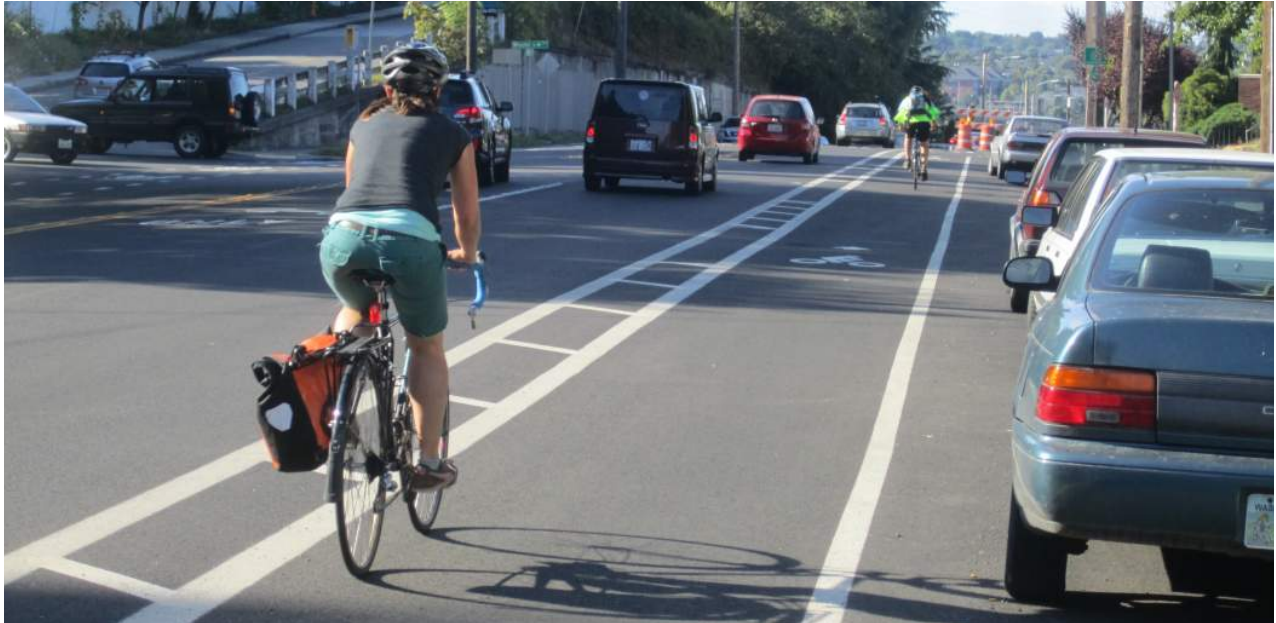
Example of Buffered Bike Lanes
