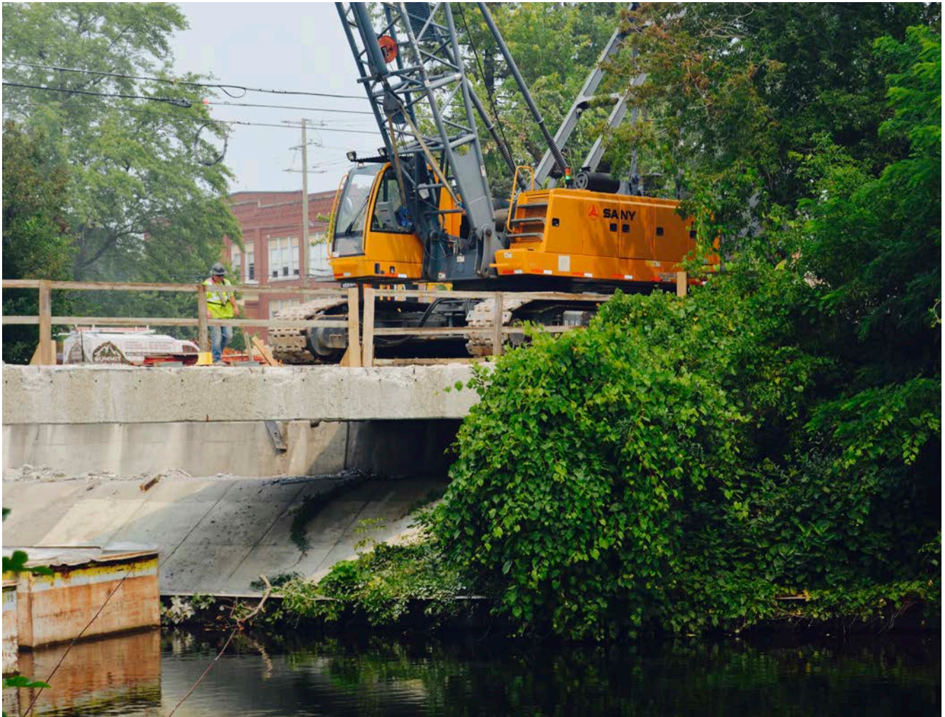
Bridge Rehabilitation. Source: City of Traverse City
