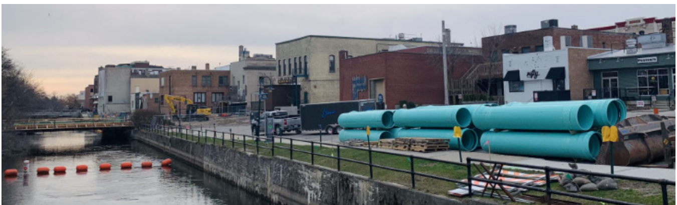
Boardman/Ottaway River Retaining Wall.
