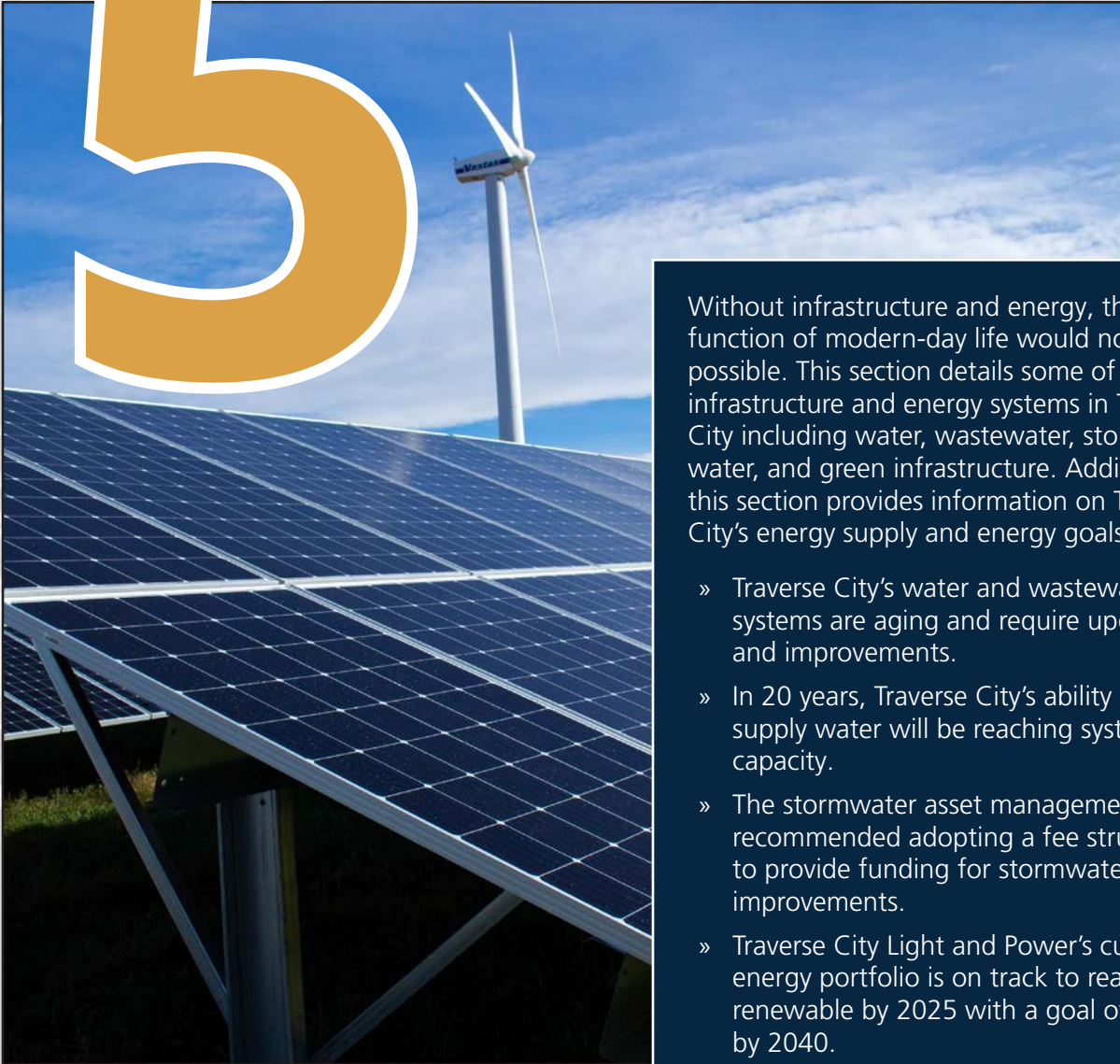
Heritage Sustainable Energy solar array on the site of the former TCLP wind turbine generator.
