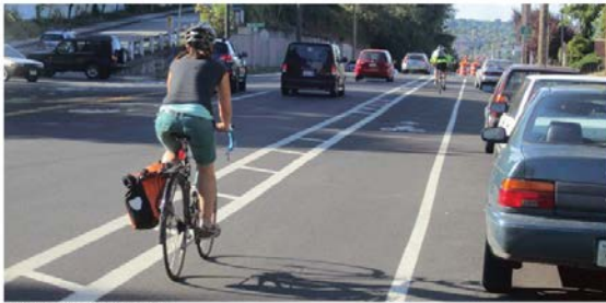
Example of Buffered Bike Lanes
