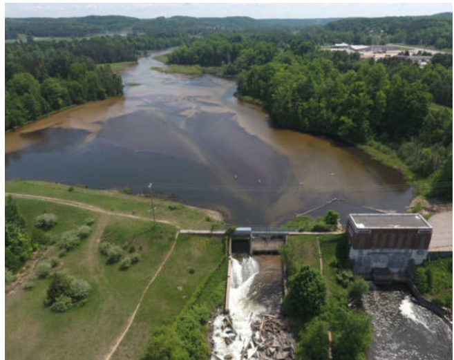
Sabin Dam prior to removal.
