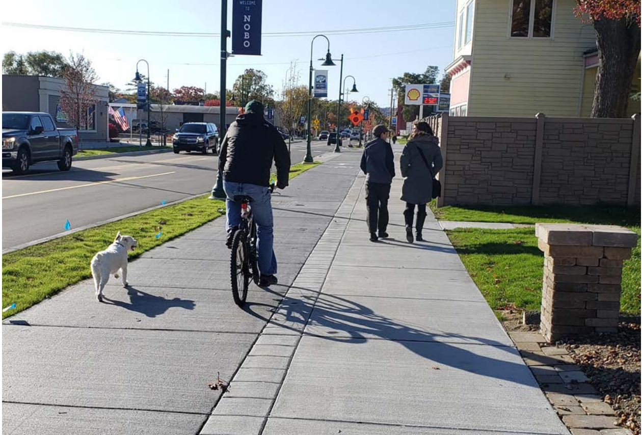
E Eighth Street Cycletrack and Sidewalk
