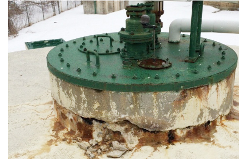
Digester #3 -cracked cap.
