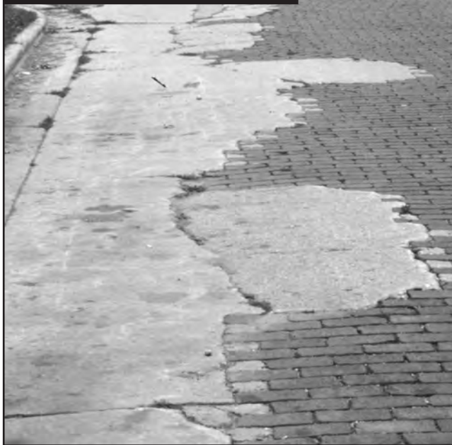
Severe brick deterioration.
