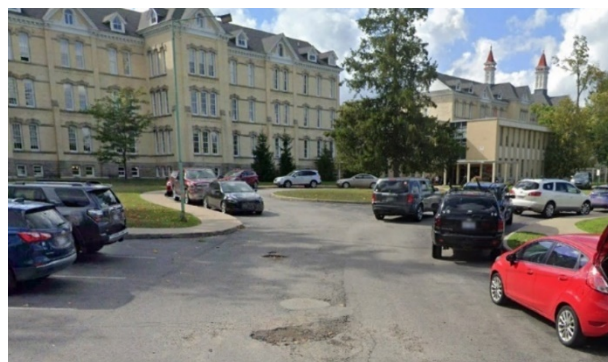
Figure 5.4: Image of Poor Pavement with Rating of 2 on 11th Street
