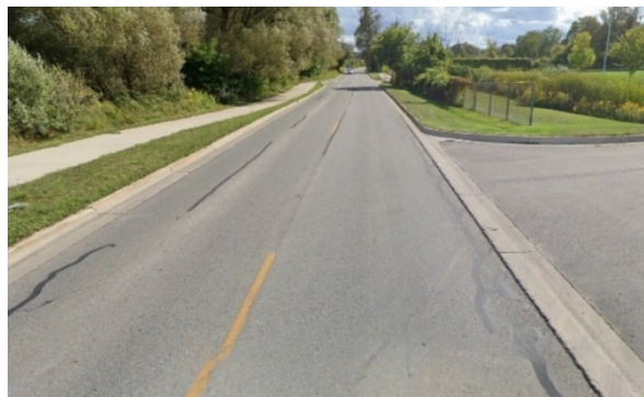
Figure 5.3: Image of Fair Pavement with Rating of 5 on Silver Drive
