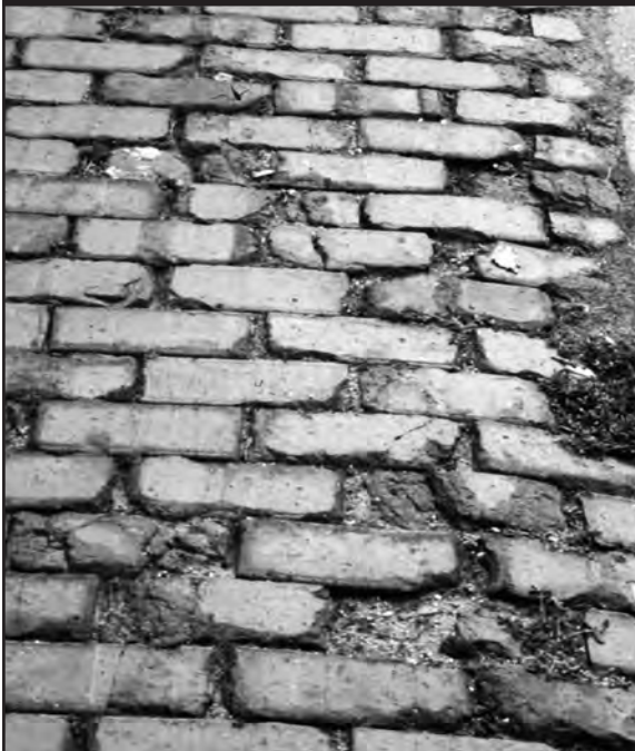
Broken bricks and rough surface over extensive area.
