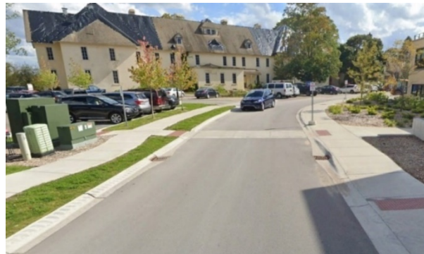
Figure 5.2: Image of Good Pavement with Rating of 9 on Red Drive
