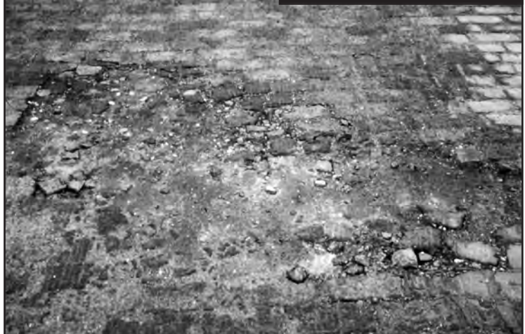
Severe brick deterioration.
