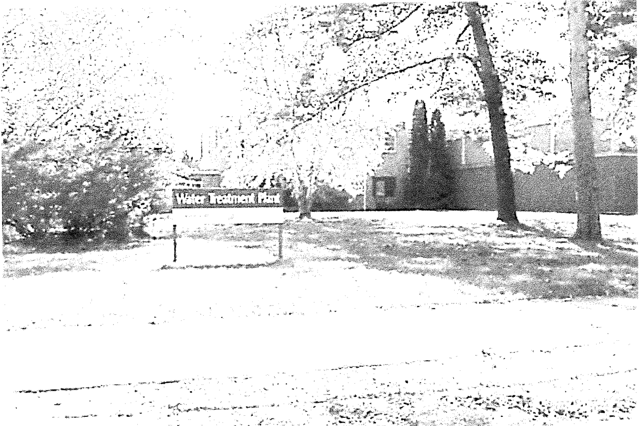
City of Traverse City Water Treatment Plant Traverse City, Michigan
