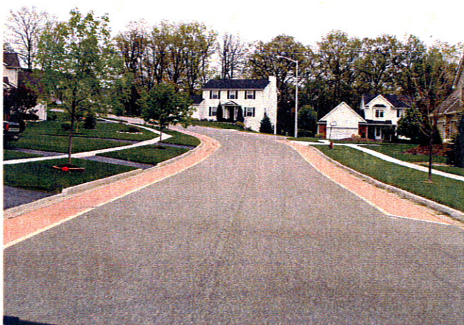
The contrasting pavement color on the Brighton, Michigan street gives an appearance of a narrower pavement. (Photo by Dan Burden)
