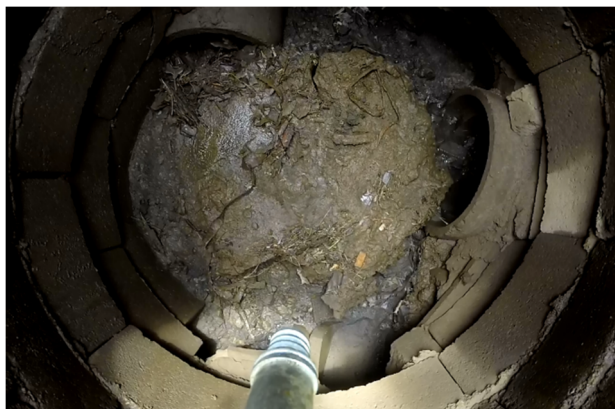
Figure 1: Manhole Deposits
