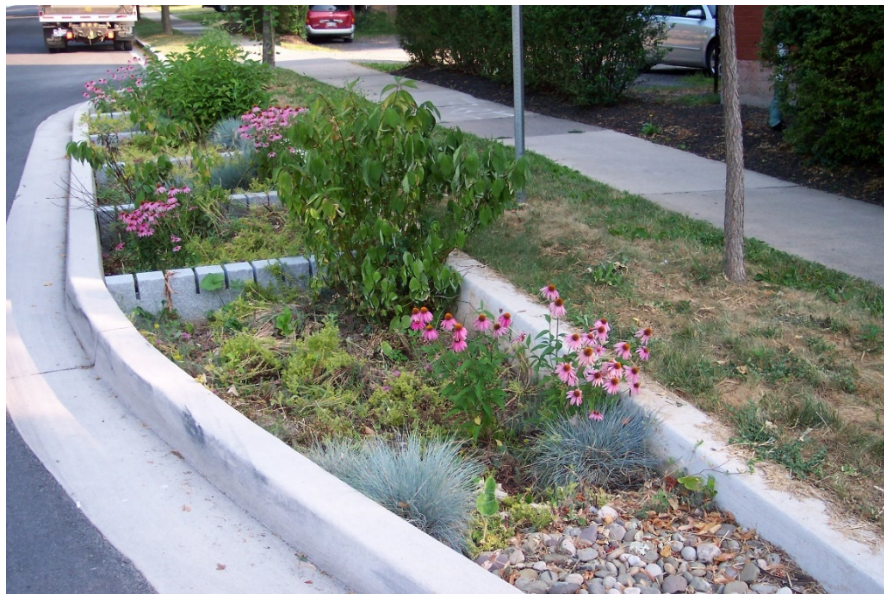
Figure C-8 and C-9: Example of BMPs within right-of-way
