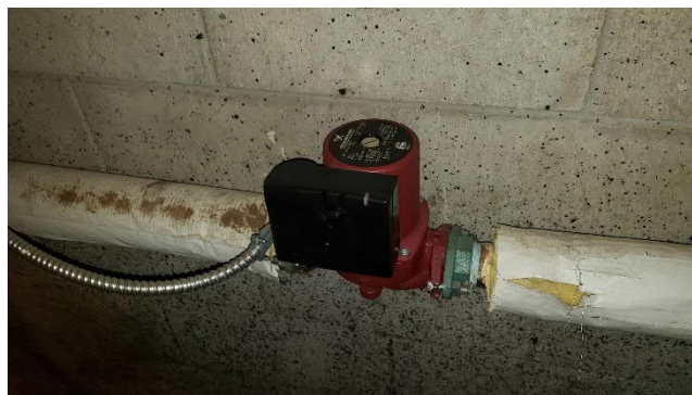
Figure M1.20 Domestic HW Recirculation Pump
