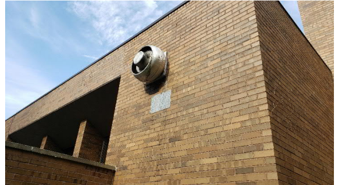
Figure M1.12 Kitchen Hood Exhaust Fan
