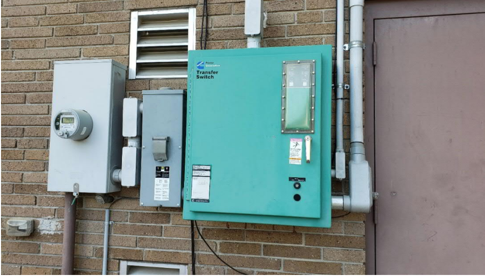
Figure E2.3 Automatic Transfer Switch (ATS) & Incoming Service Equipment
