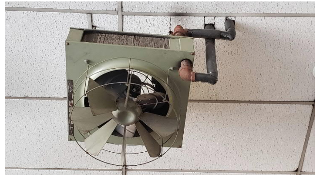
Figure M2.2 Apparatus Bay Unit Heater (typical of 2)
