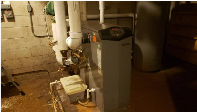
Figure M1.1 Existing Lochinvar Boiler (in basement)
