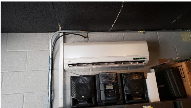
Figure M2.7 Mini-Split A/C Unit (indoor evaporator)
