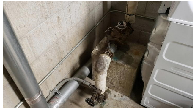
Figure M1.18 Metered Domestic Water Service (2" with BFP)
