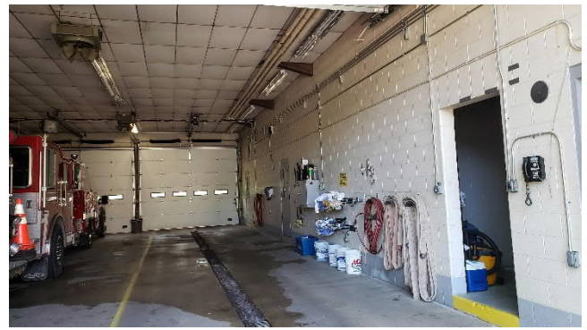
Figure M2.12 Apparatus Bay (no vehicle exhaust capture)
