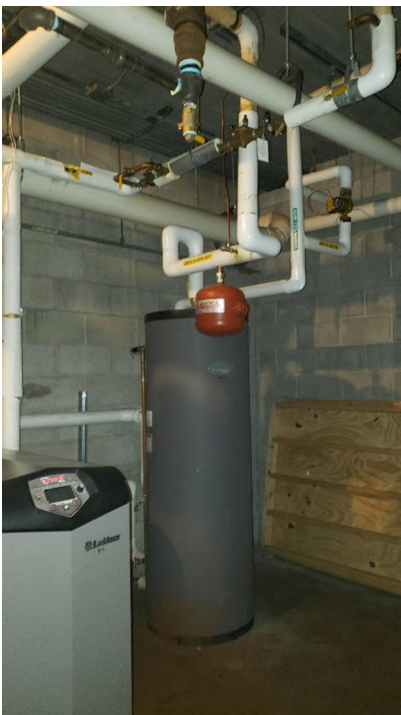
Figure M1.19 Domestic HW Storage Tank
