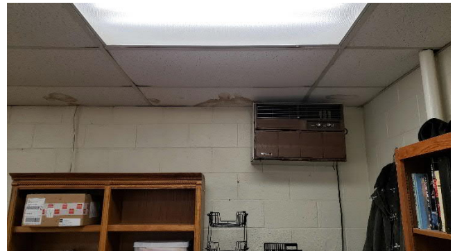
Figure M1.8 Thru-Wall A/C Unit
