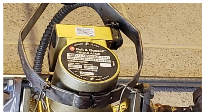
Figure M2.16 Domestic Hot Water Recirculator
