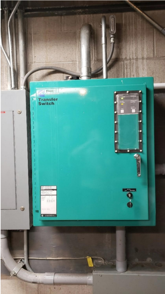
Figure E1.3 Automatic Transfer Switch (ATS)
