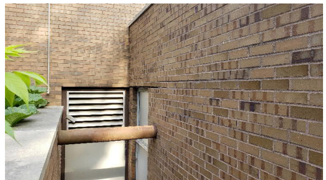
Figure M1.10 Fresh Air Intake Louver for AHU
