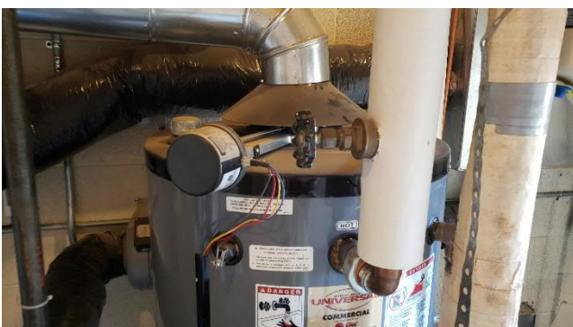
Figure M2.15 Domestic Water Heater
