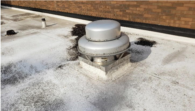
Figure M1.11 Rooftop Exhaust Fan
