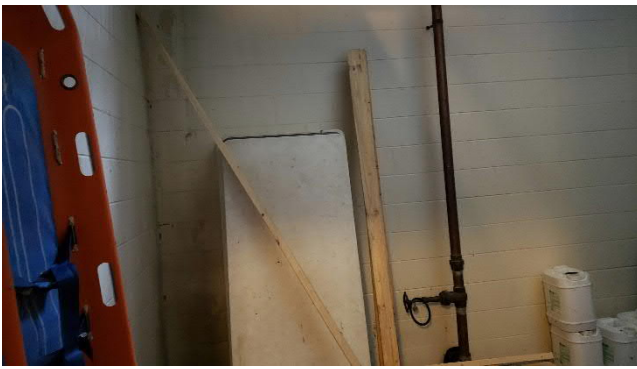
Figure M1.17 Unmetered Domestic Water Service (2.5")
