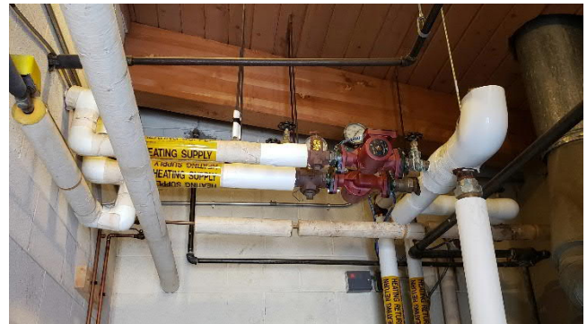
Figure M2.4 Heater System Zone Pumps
