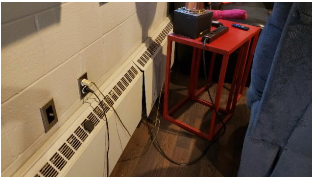
Figure M2.3 Typical Perimeter Heating Unit
