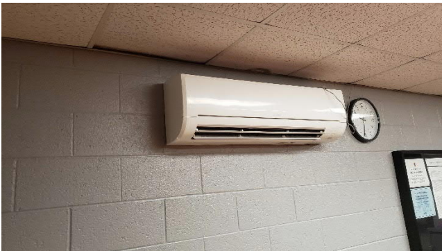
Figure M1.7 Mini-Split A/C Unit (indoor evaporator)
