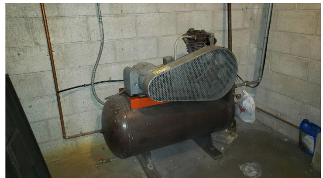
Figure M1.16 Air Compressor for Temperature Controls
