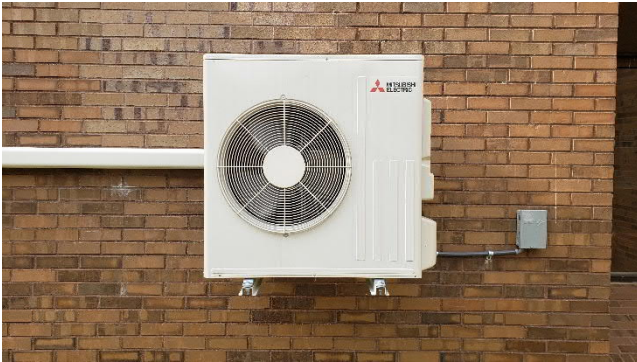
Figure M1.5 Mini-Split A/C Unit (outdoor condenser)
