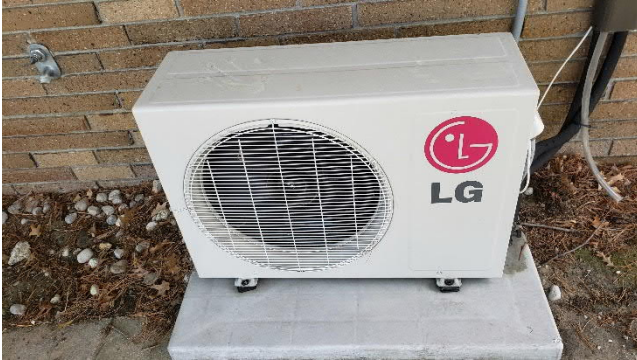
Figure M2.5 Mini-Split A/C Unit (outdoor condenser)
