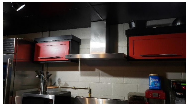
Figure M2.10 Kitchen Range Exhaust Hood
