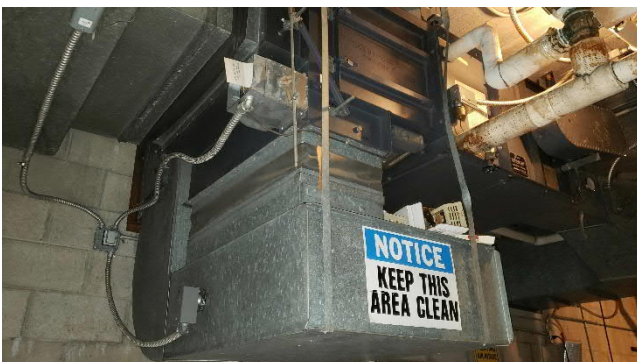
Figure M1.9 Heating & Ventilation AHU (in basement)
