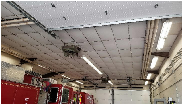
Figure M2.11 Apparatus Bay (no gas detection or exhaust system)
