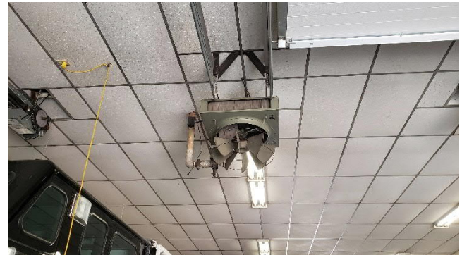
Figure M1.2 Apparatus Bay Unit Heater (typical of 4)
