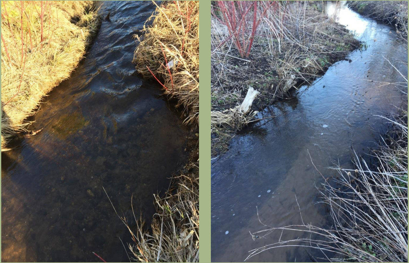
Figure 24. Conditions of installed riffle cobble on two designed riffles on Tributary A daylighting project. On the left, visible cobble; on the right no cobble visible due to sand deposition.
