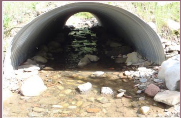
Figure 21. Example of Culvert bottom roughening (USFS photo)
