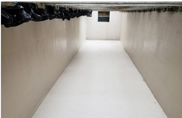
Membrane replacement – train 8 newly coated.
