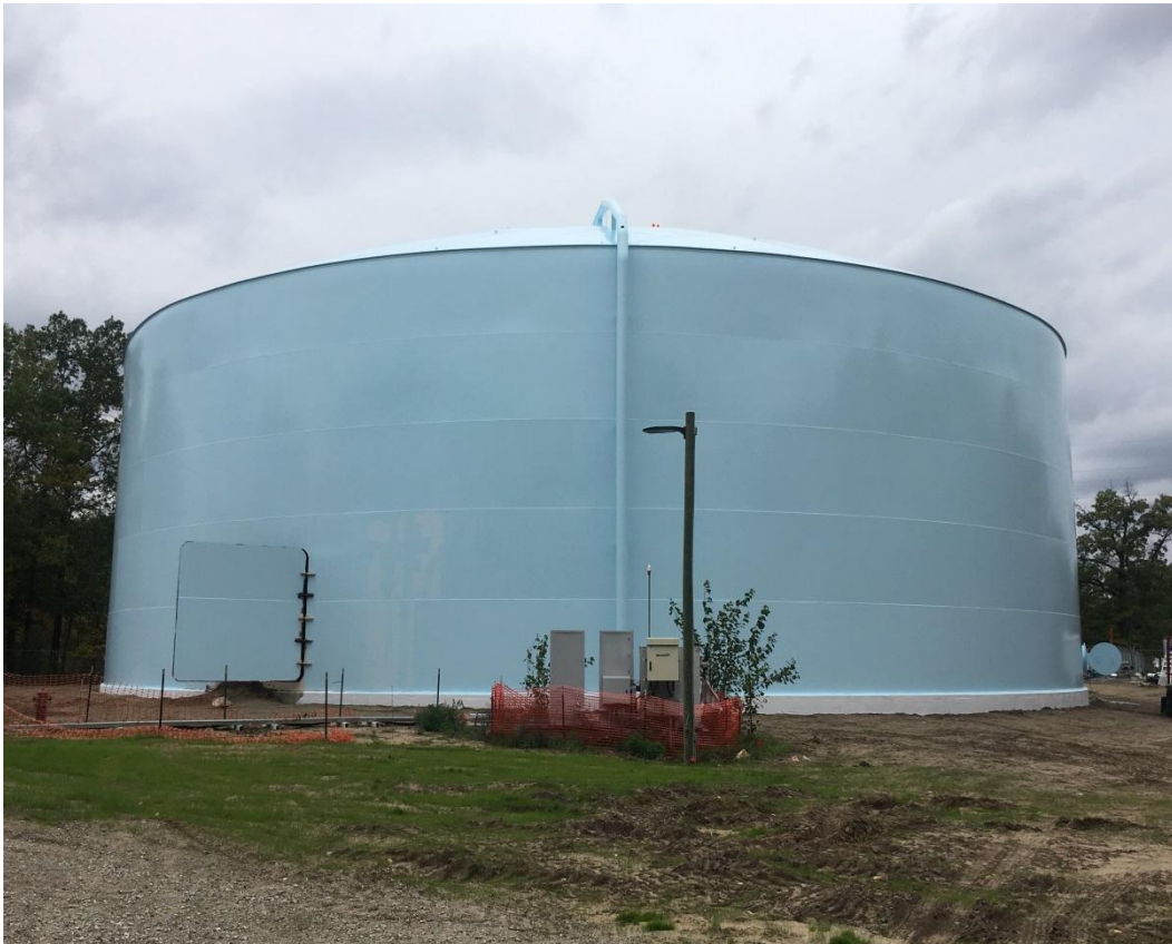
Barlow 4 MG Water Reservoir Rehabilitation Project (Completed in 2020)
