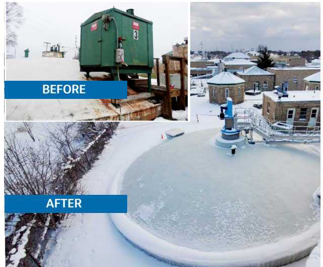
Digester 3 rehabilitation – exterior.
