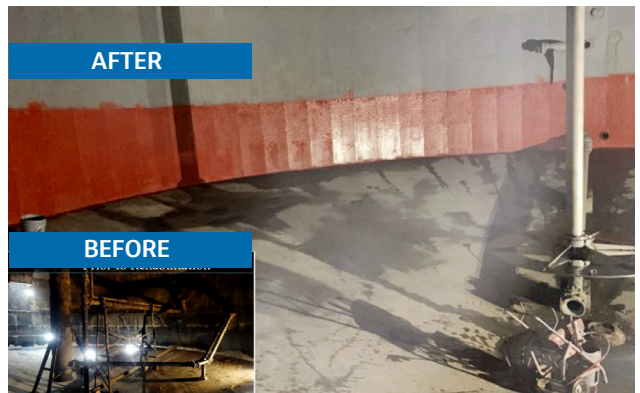
Digester 3 rehabilitation – interior.
