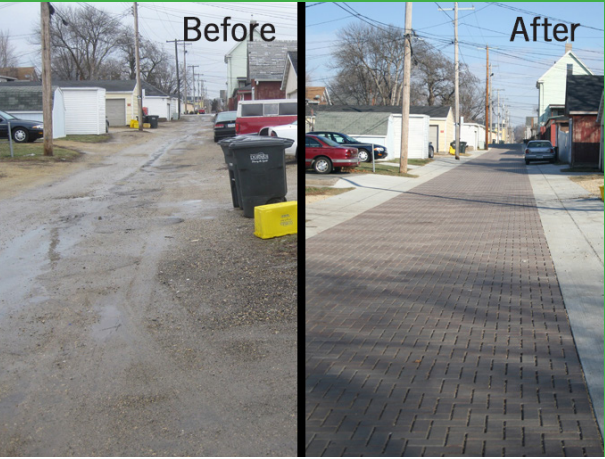
Green Alley Installation in Dubuque, Iowa
