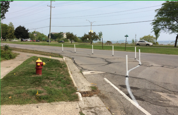
Temporary Curb Extension at Monroe and Bay Intersection
