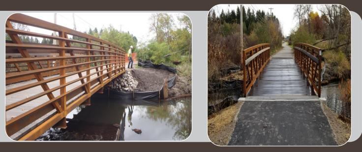
Replaced existing concrete box culverts with clear span pedestrian bridges in two locations on Kids Creek. This project is funded through a grant obtained by the Watershed Center Grand Traverse. Elmer's Crane & Dozer was hired to complete the work. One location is the old railroad grade between Division St and Silver Dr and was completed in conjunction with a paved path that is part of the Safe Routes to School Project.
