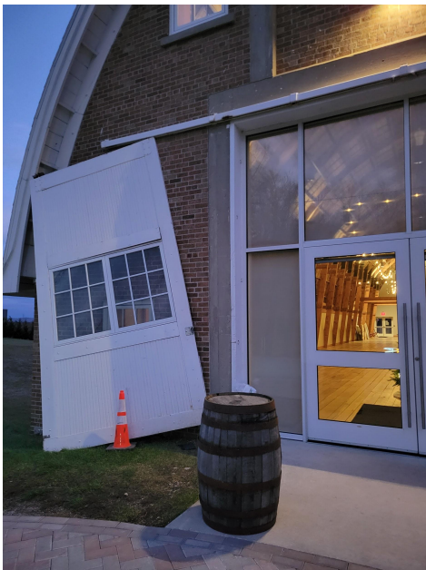
Main entrance door damage from windstorm.
