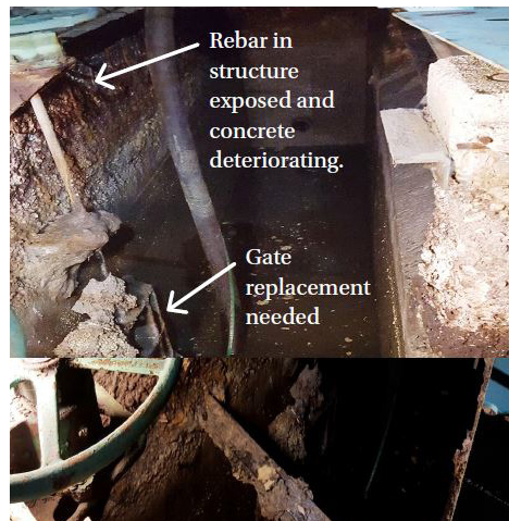
East grit effluent channel discharging to primary header.
