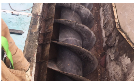
General condition of screw pumps 2 and 3.
