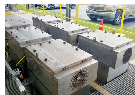
After modules were lifted out of the flood zone.
