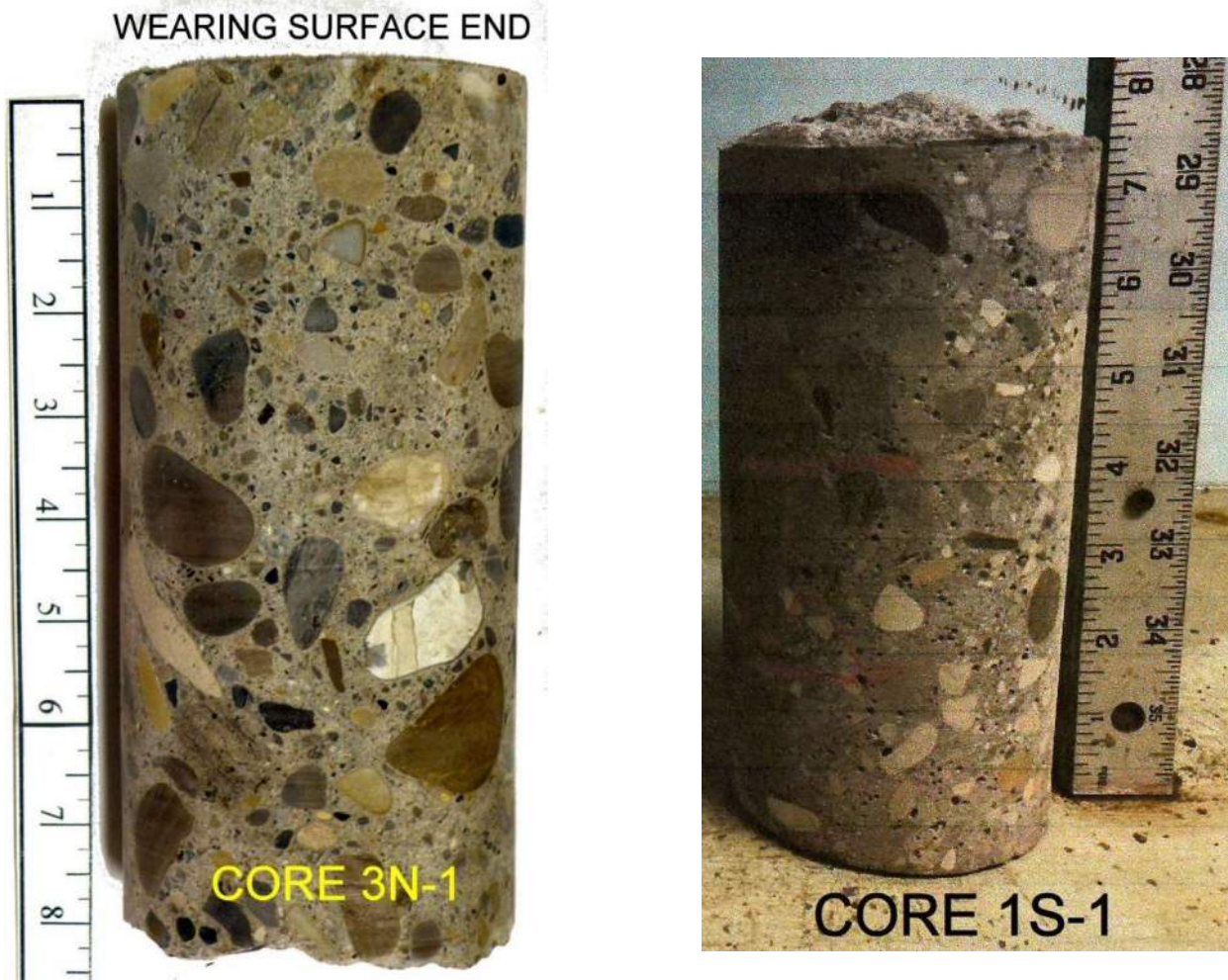
Figure 2. Cores 3N-1 and 1S-1 provided for the petrographic examination. Core 3N-1 was received intact. Core 1S-1 was tested for compressive strength at G2, following which the fracture pieces were provided for the petrographic examination.
