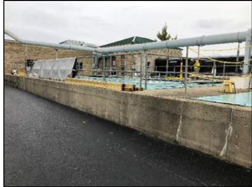
Photo 9- Repairs along north wall of Tank 4N
