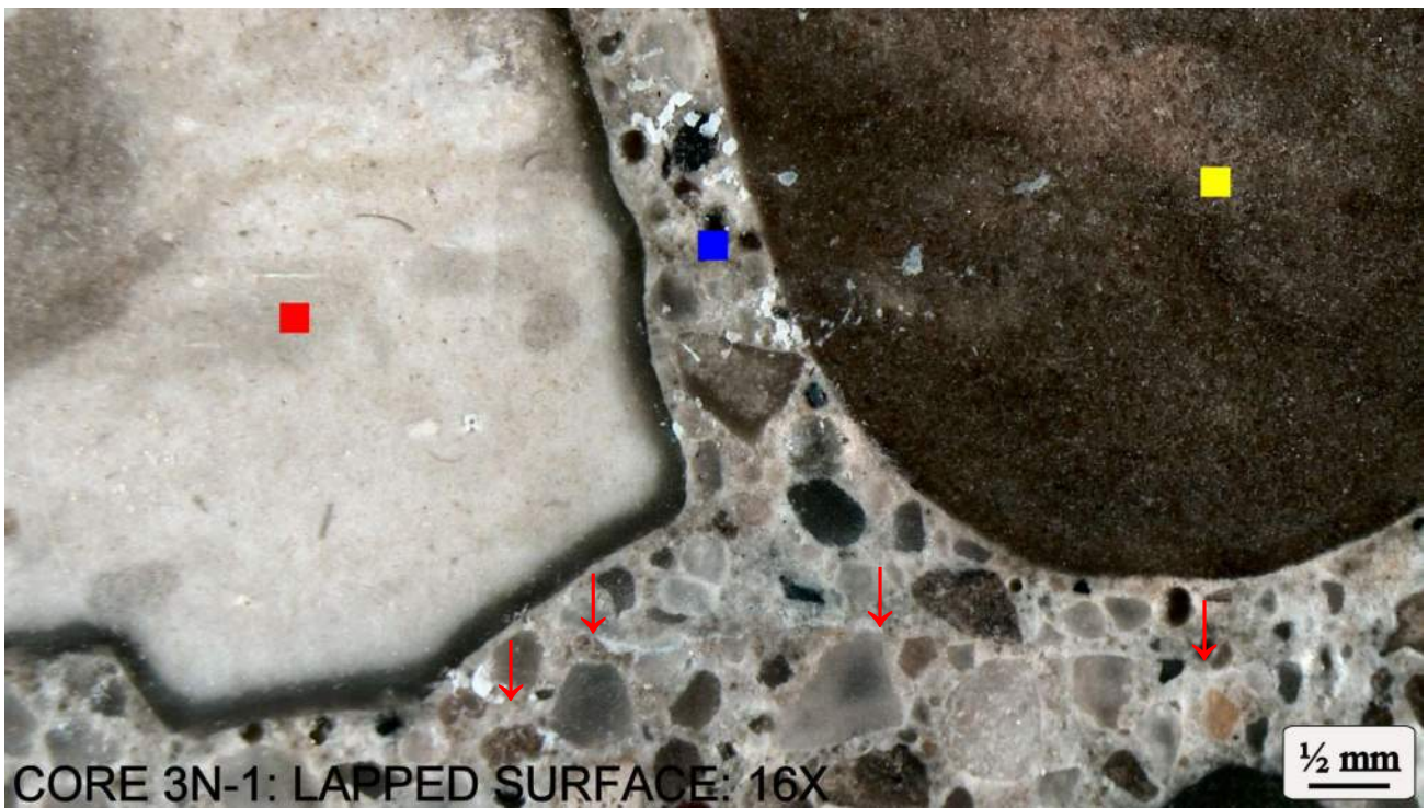
Figure 13. These are photographs, taken at a magnification of 7X and 16X, on a lapped surface of Core 3N-1. The red arrows point to ASR-related microcracks. Features of interest are discussed below.
