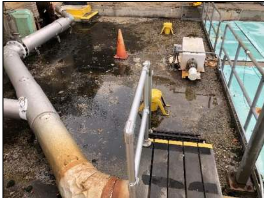
Photo 5- Standing water across top slab on west end of Tanks 1 and 2S
