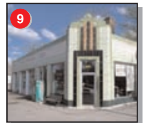
9 Max's Super Service Station, 501 South Union Street
