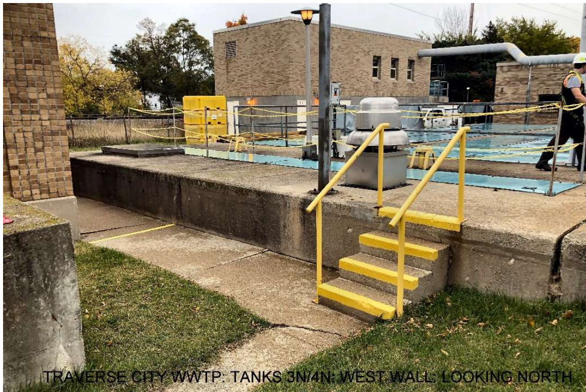
Figure 1. Views of the Traverse City WWTW facility in October 2014. The top view shows the tanks labeled 1S and 2S. Core 1S-1 was taken from the vertical wall separating Chamber 1S from 2S (1930s construction). The bottom view shows Tanks 3N and 4N. Core 3N-1 was taken from Tank 3N, which was constructed in the 1960s.
