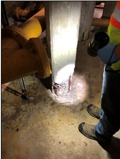
Photo 10- Deteriorated concrete w/ exposed reinforcement at column base
