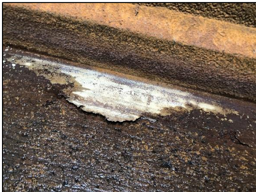
Photo 3- Concrete slab beneath hardened sludge
