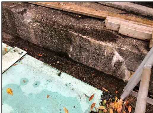
Photo 8- Deterioration along grit chamber walls
