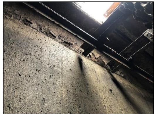
Photo 7- Coating failure at waterline
